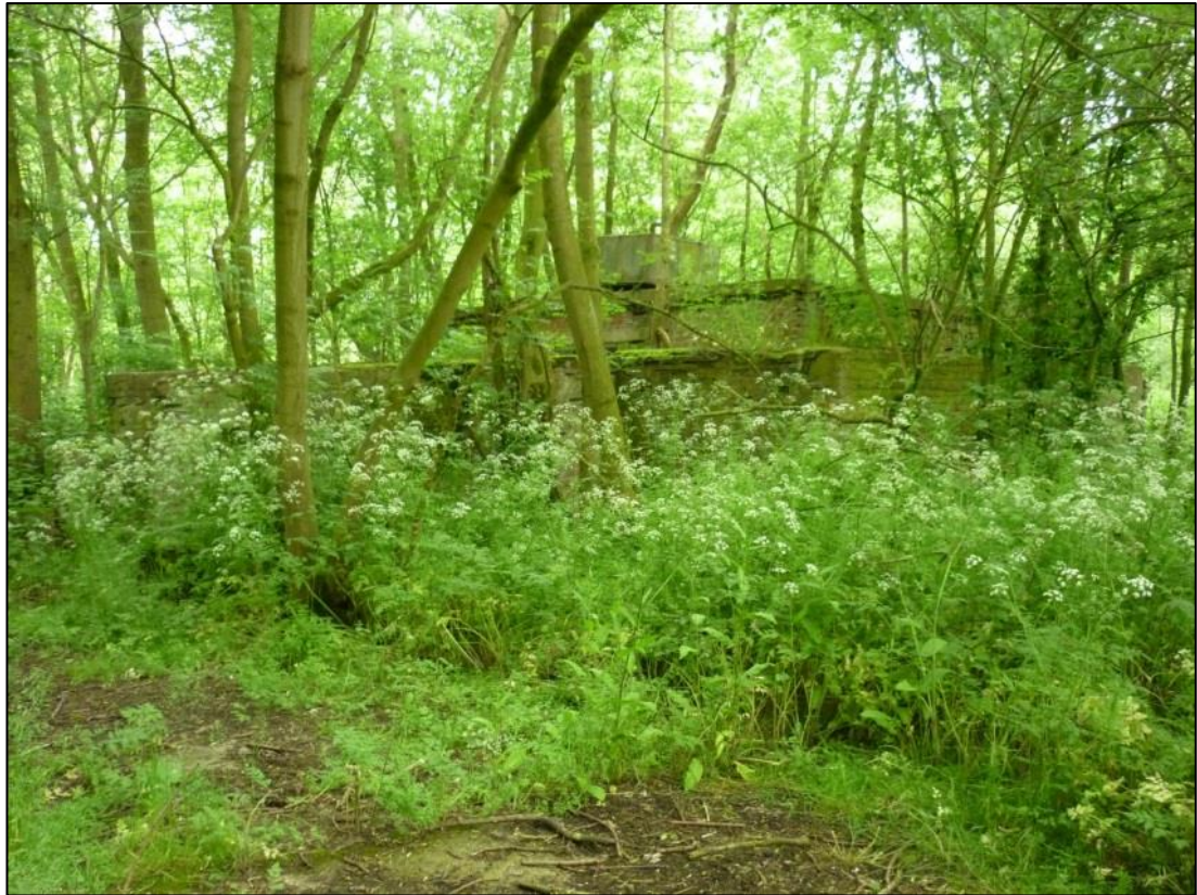
Figure 1: Magazine at the Office of Strategic Service's (OSS) 'Area H'. The extensive vegetation growth within this facility has resulted in the rapid deterioration of the surviving structures. 21
