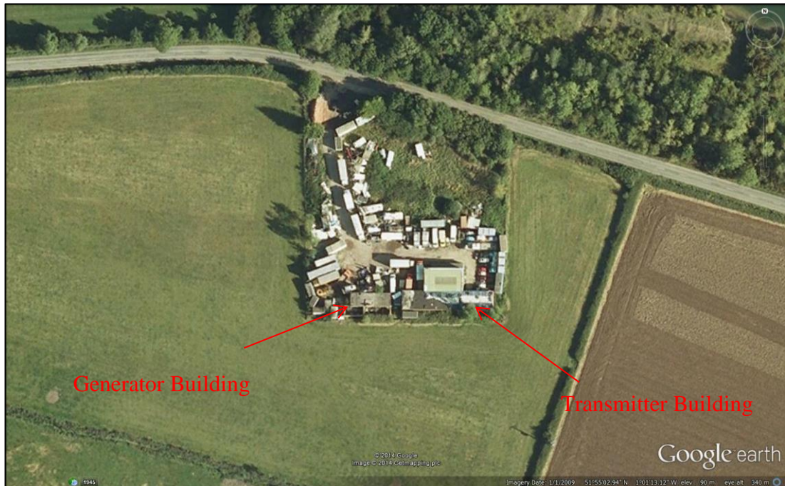
Figure 107: Station 53a's new transmitter at Charndon. Based on the design of Godington, this facility was constructed to enable SOE to keep up with increasing operational demands for wireless communications. 46
