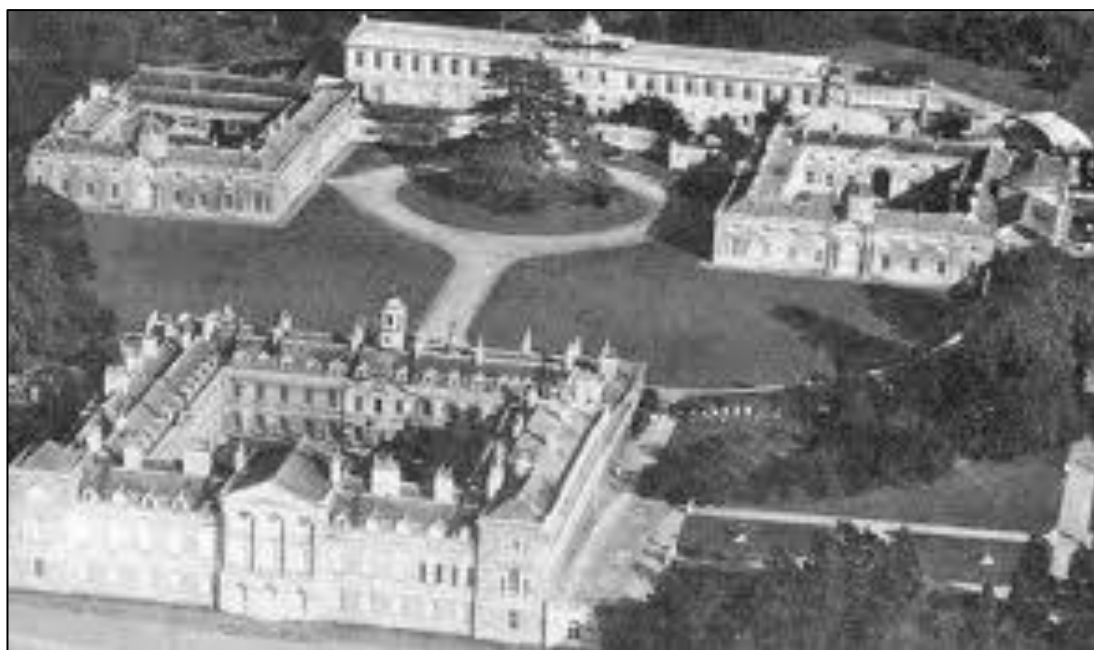
Figure 9: The Riding School, the linear building at the back of the photograph, at Woburn Abbey. At the outbreak of the Second World War, Department EH relocated to this property.
