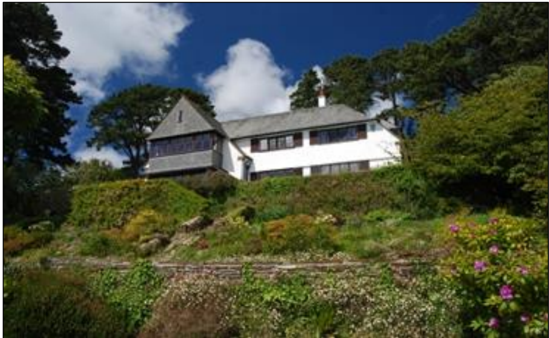
Figure 82: Ridifarne, home to the shore establishment of the Helford Flotilla. Located next to a pool in the estuary, this location allowed SOE's ships to remain afloat at all tides.
