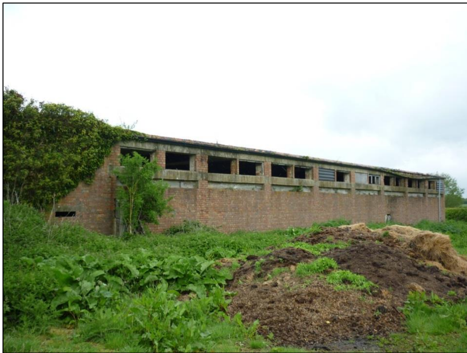
Figure 103: The transmitter building of SOE's Station 53b at Godington. Structural evidence indicates that the complex was constructed in two phases. 34
