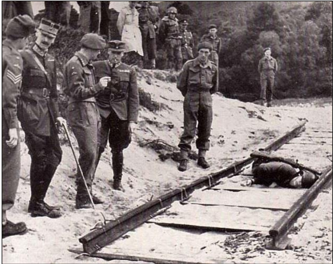
Figure 19: Industrial sabotage and wireless operation were some of the specialist topics taught to students at SOE's STSs. Within the grounds of several of SOE's STSs, railway track was laid so that the students could practice demolition techniques. 97
