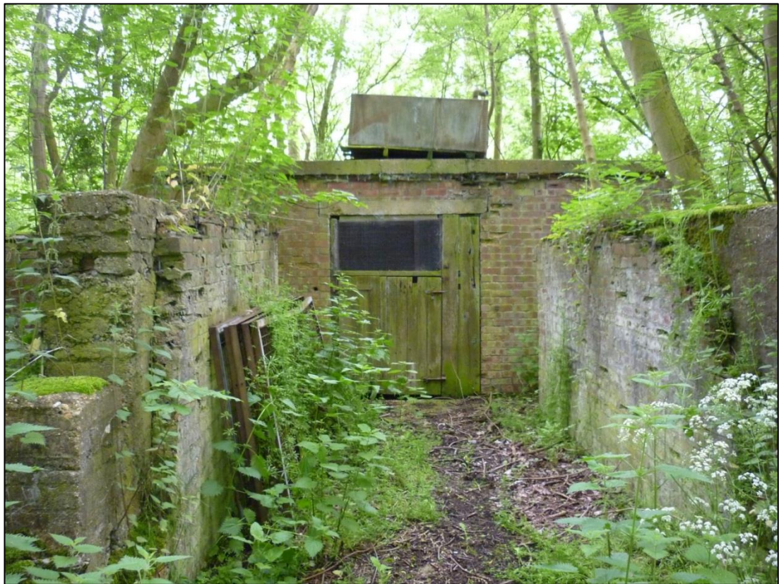
Figure 78: One of the magazines at Area H. Since the end of the Second World War, all of SOE’s structures at Gaynes Hall have been demolished and replaced with a prison. As nothing survives there, Area H is a valuable analogy for visualising SOE’s facility. 96
