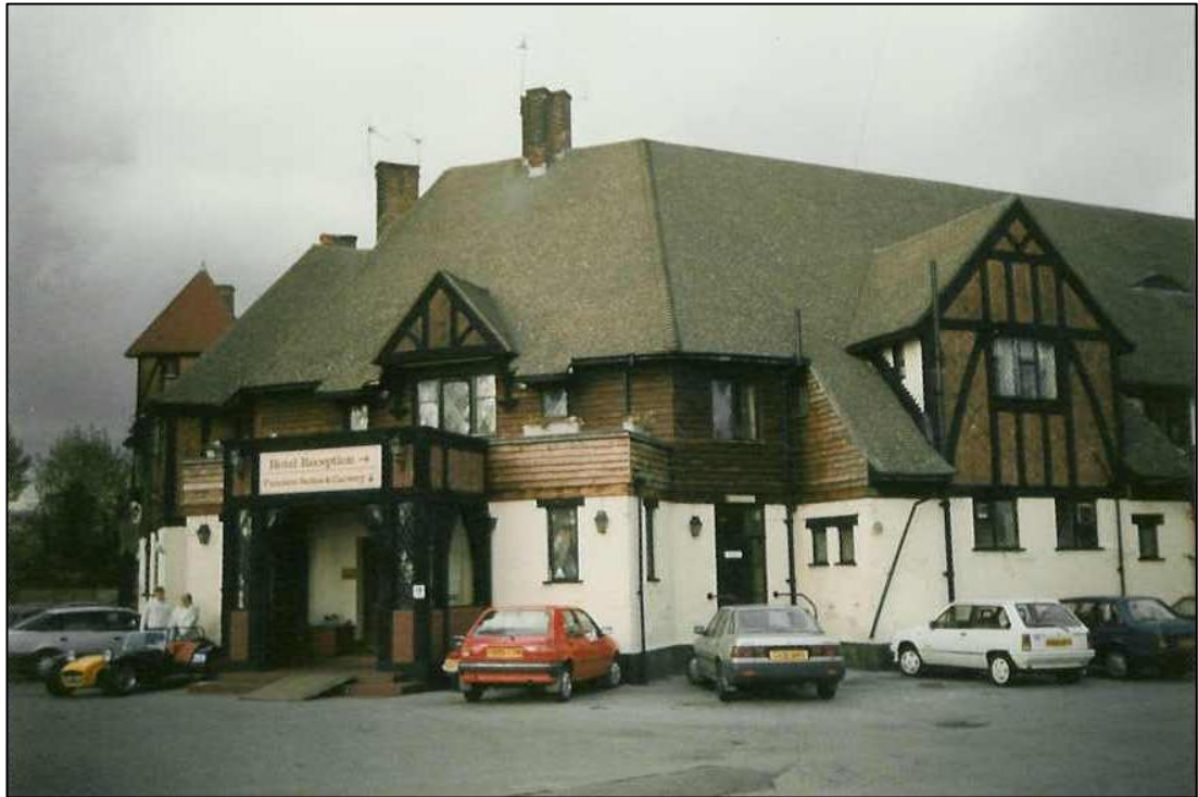
Figure 58: The Thatched Barn, located on the Barnett bypass. In June 1942, SOE relocated their Camouflage Section from the Victoria and Albert Museum to this new accommodation.
