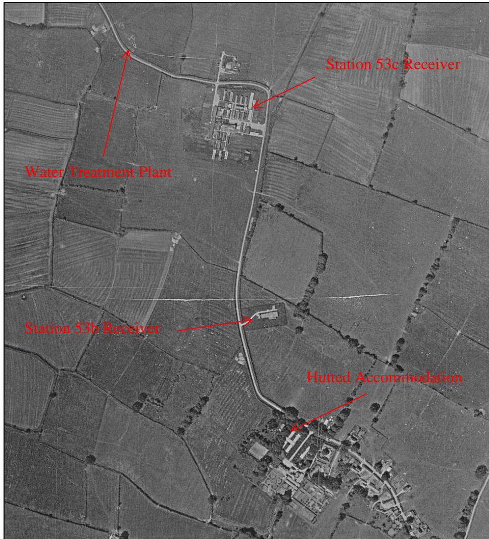
Figure 101: (centre) The receiver of SOE's first purpose built Home Station, Station 53b. Originally, the structure was square which indicates that an expansion of this facility occurred sometime after construction. This probably coincided with the two phases of construction at Godington. 31
