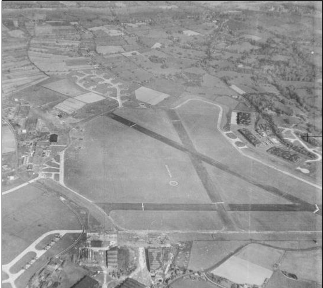
Figure 21: RAF Ringway, 1946. This airfield was of a typical design for the Second World War. 111
