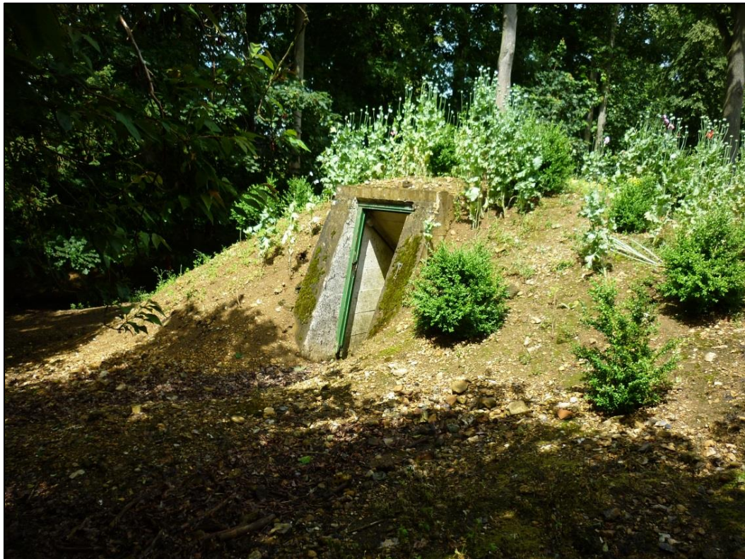
Figure 35: Entrance to one of the underground structures at Frogmore Hall. These structures were approximately 2m by 20m and constructed of poured concrete. 168
