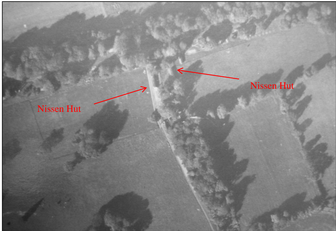
Figure 23: Aerial photograph of Gorhambury, Hertfordshire, taken in 1946. From aerial photographic analysis, it appears that it was uncommon for SOE to construct buildings at their STSs. At sites where SOE did erect structures, they appear in woodland at a distance from the main property. Further ground based survey is, therefore, necessary to determine the extent of SOE's building programme at STSs. 123
