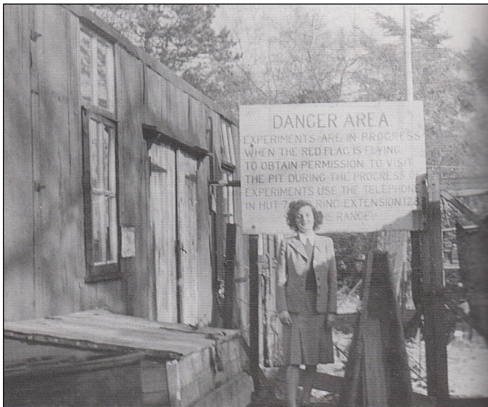
Figure 42: Hut in the grounds of The Frythe. The first structures constructed at this facility were single-storey, prefabricated wooden huts roofed with felt. 35
