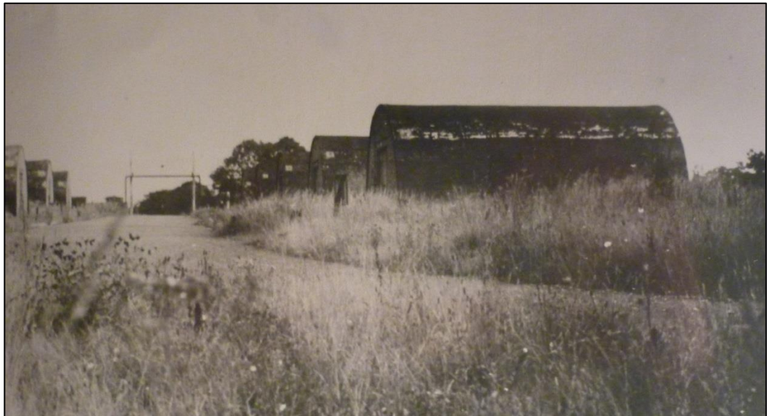
Figure 71: Storage facilities at Aston House. Located to the south-west of the main house, these structures are believed to be for the storage of incendiary devices. In the background, an overhead hot steam pipe can be observed. Heat was produced in the generator building and then piped round the facility. 66
