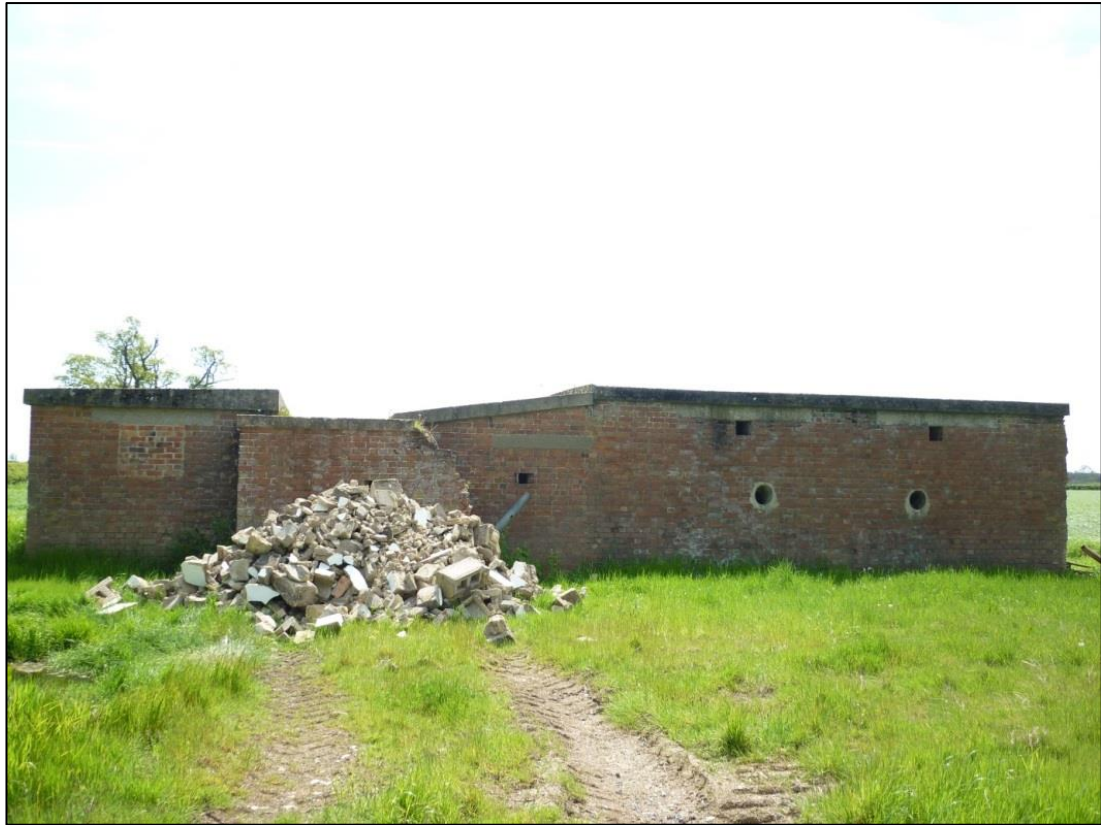
Figure 99: SOE's first transmitter at Charndon. The structure to the left was the first transmitter building; the extension to the right was a later addition. Structural analysis indicates that there was at least three phases of construction. 26
